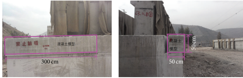
FIGURE 3: Preparation of the concrete beam specimen.
