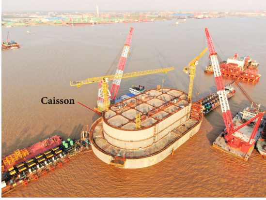
FIGURE 2: Caisson under construction.
