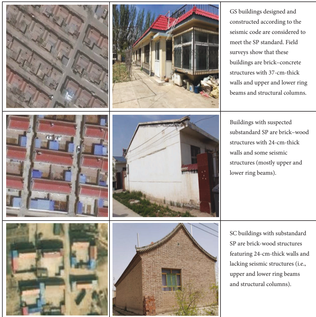
FIGURE 4: Typical buildings in rural and RUF areas.
