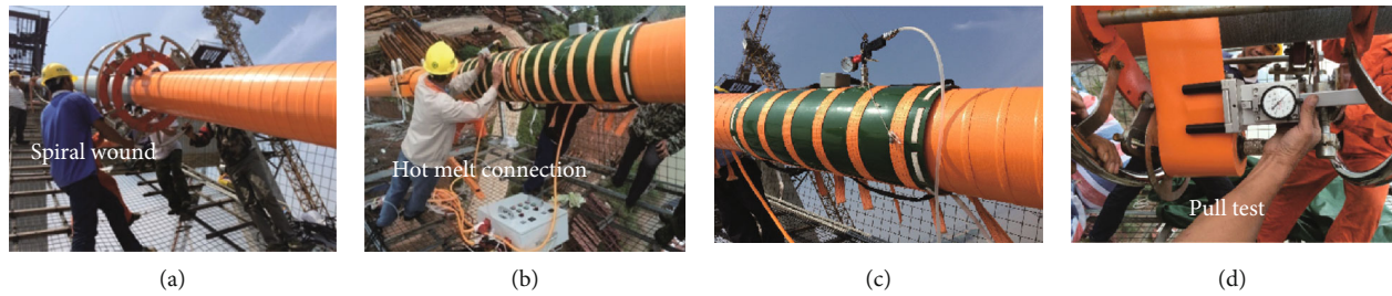
FIGURE 4: The construction process of winding and heating pressure vulcanization.
