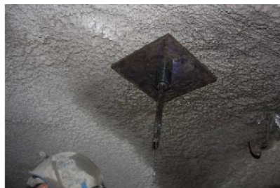
Middle (before grouting)
