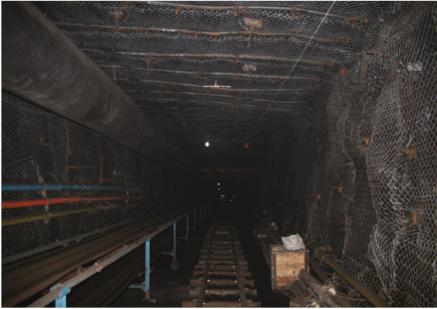
FIGURE 18: Good result of the support scheme.
