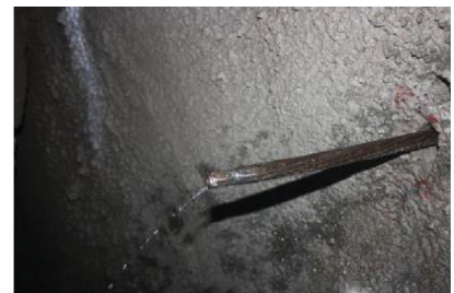
Right (before grouting)
