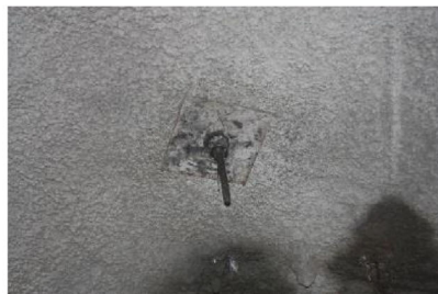
Middle (after grouting)
