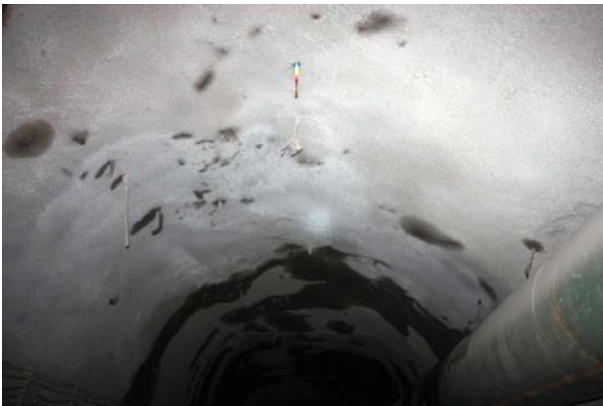
FIGURE 2: Roadway appearance (without anchor cable).
