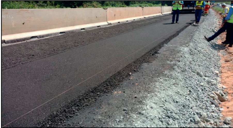
FIGURE 7: Construction of the first layer of the cold recycled mixture.
