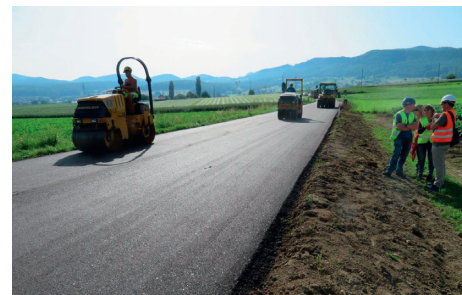
FIGURE 17: Test section with RAP material at the end of compaction.
