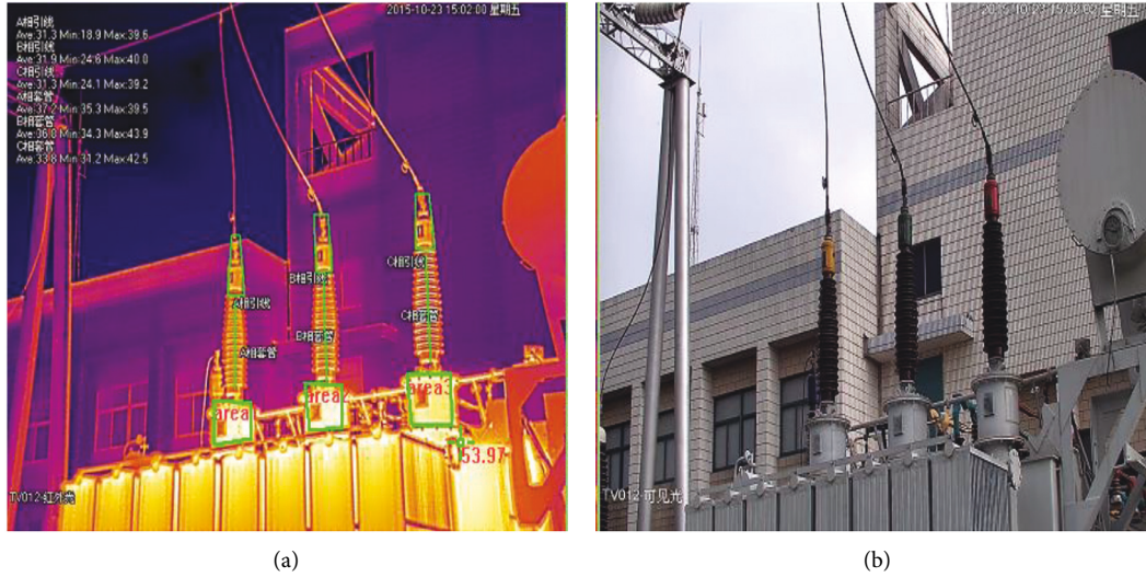
FIGURE 7: Substation equipment diagram. (a) Infrared imaging diagram. (b) Substation equipment diagram of substation equipment under visible light.
