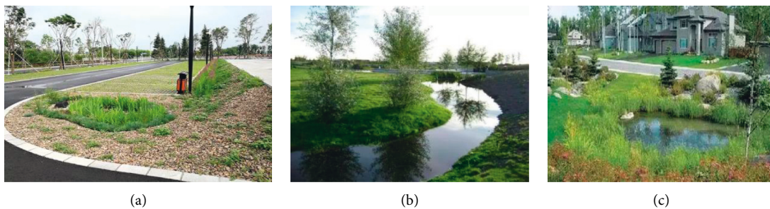
FIGURE 11: Typical green stormwater infrastructure. (a) is the decentralized control measures at the source—concave green space; (b) is the transportation measure—shallow ditch with vegetation; (c) is the centralized control measure at the end—ecological pool.
