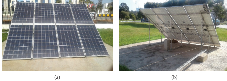
FIGURE 3: ENSET School PV system. (a) The panels' orientation. (b) The panels' structure.
