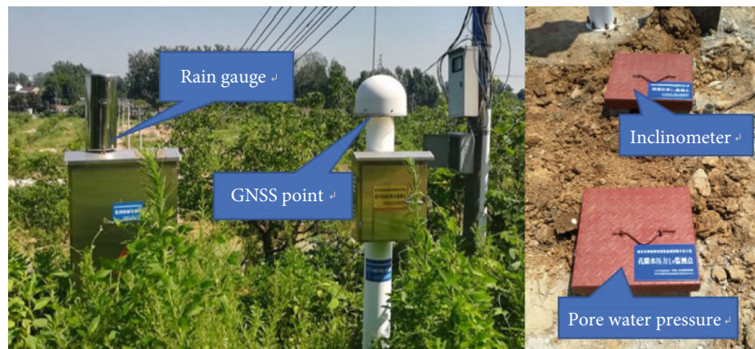
FIGURE 3: Monitoring instruments on the landslide.
