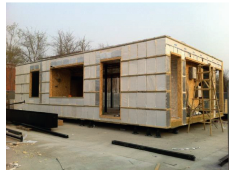
FIGURE 5: Building's exterior wall with HIPs employed during the building process (source: authors' own data).
