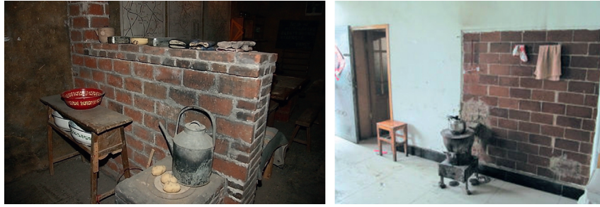
FIGURE 1: Traditional Chinese heated walls commonly used in northern China (photograph: left: http://www.huitu.com/photo/show/20121107/154758101200.html ; right: http://news.163.com/14/1014/10/A8GSP17D00014AED_mobile.html ).
