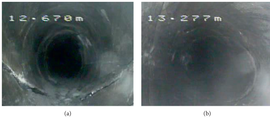
FIGURE 9: Separation of the roof. (a) No. 1 borehole-separation (b) No. 2 borehole-separation.
