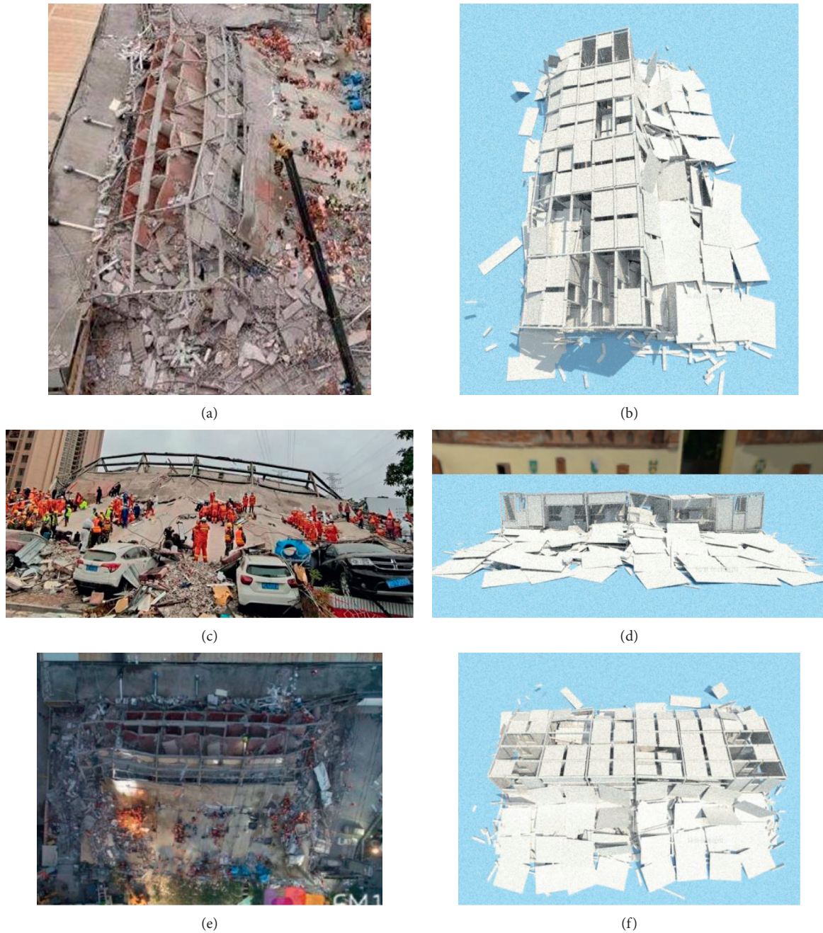
FIGURE 12: Comparison between actual physical collapse wreckage and simulated virtual wreckage. (a) Actual collapse scenario (side view); (b) simulated collapse scenario (side view); (c) actual collapse scenario (front view); (d) simulated collapse scenario (front view); (e) actual collapse scenario (top view); (f) simulated collapse scenario (top view).
