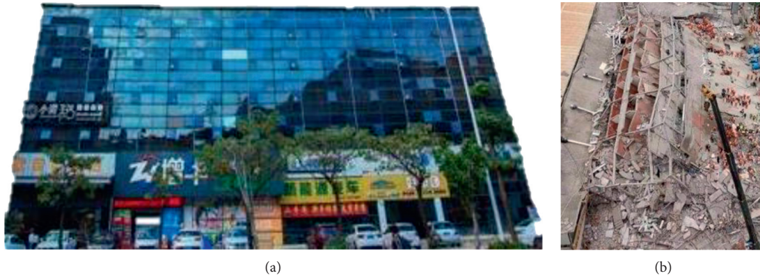
FIGURE 2: Hotel building before and after the collapse. (a) The hotel building before collapse (the hotel name is anonymous). (b) Ruin after the collapse.
