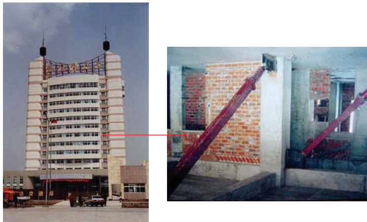
Figure 9: Viscoelastic dampers in Suqian Communication Building.
