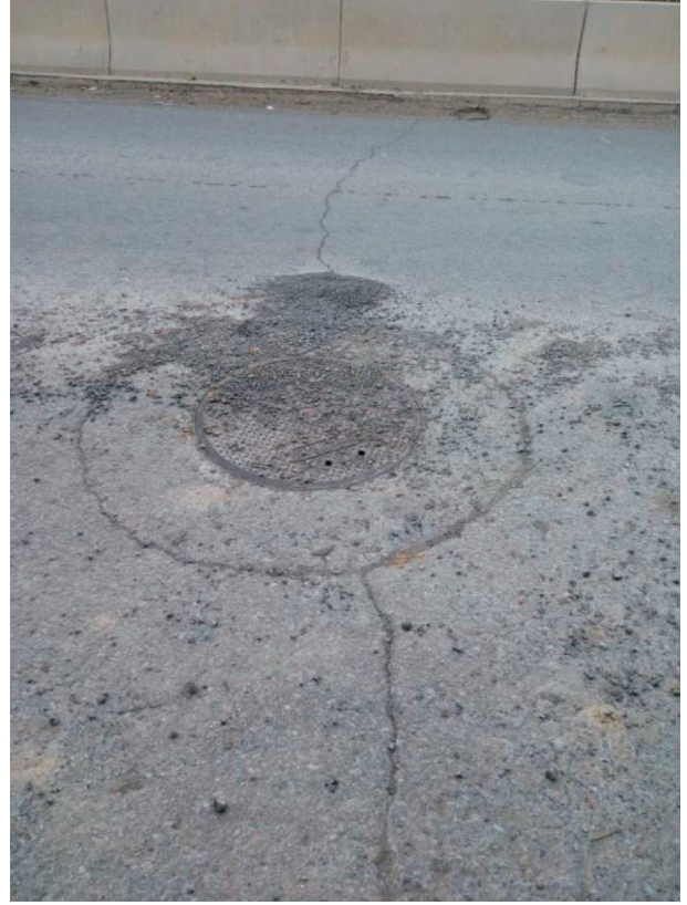
FIGURE 1: Crack of asphalt pavement structure.
