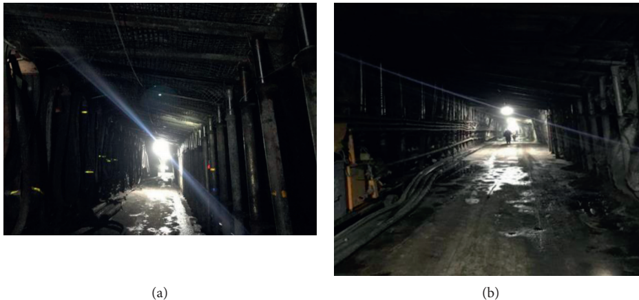
FIGURE 12: Effects on the roadway with 50 and 100 m of working face advancement. (a) 50 m of advancement and (b) 100 m of advancement.
