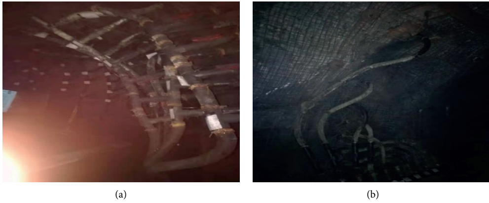
FIGURE 2: Inclination test site. (a) Drilling site at the early stage of treatment. (b) Drilling at the later stage of treatment.
