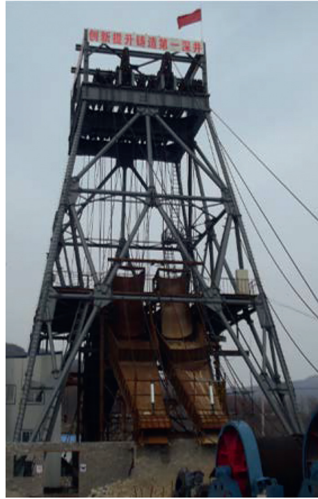
FIGURE 2: The working condition of sinking headframe in the field.
