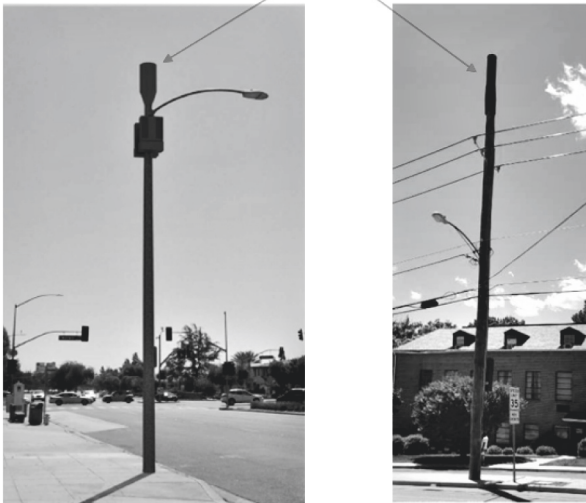
FIGURE 12: Microcell towers (these for 4G, but a lot more for 5G). (non-copyrighted material from FCC-related filings [91]).
