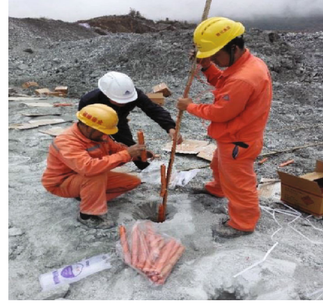
FIGURE 4: Air interval charging.
