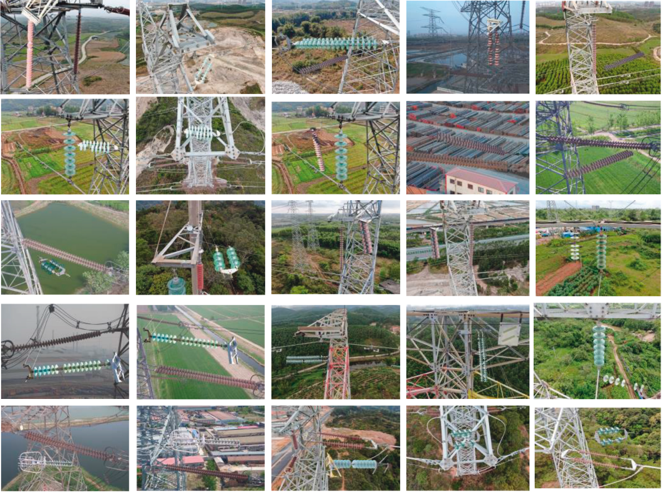
FIGURE 4: Parts of generated defective insulator images.
