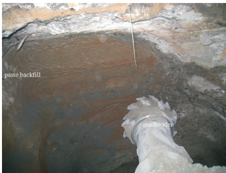
FIGURE 7: Excavating tunnel in paste backfill.
