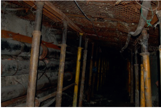
FIGURE 10: Roadway at 160 m after working face.
