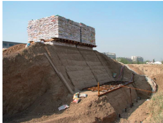
FIGURE 8: Multi-stage loading on the top of the landslide model.
