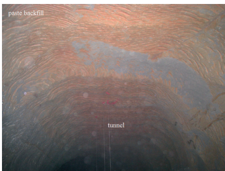
FIGURE 8: Completed tunnel in paste backfill.
