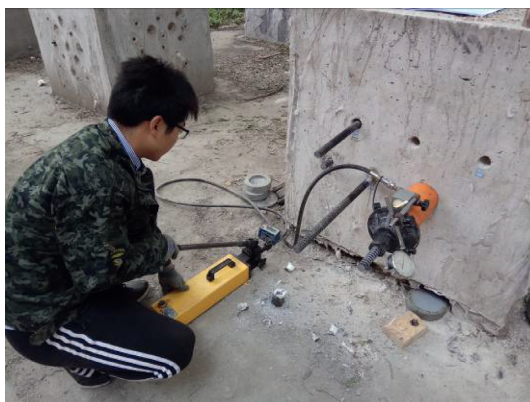
FIGURE 7: Pull-out test of different bolts.
