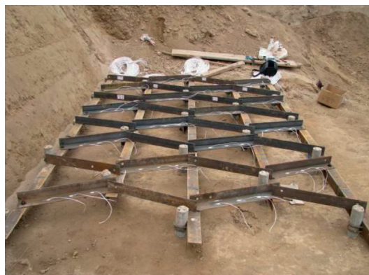
FIGURE 5: The connecting beam on the top of micropiles.
