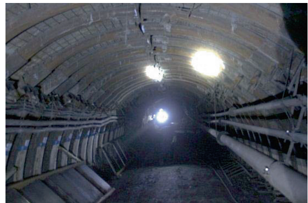
FIGURE 11: 1412 Roadway after support.
