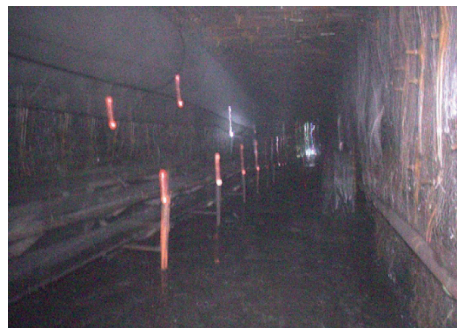
FIGURE 23: The stable environment of surrounding rock in 8103 headgate.
