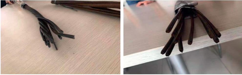
FIGURE 2: Cable breakage of No. 3 exploration roadway.
