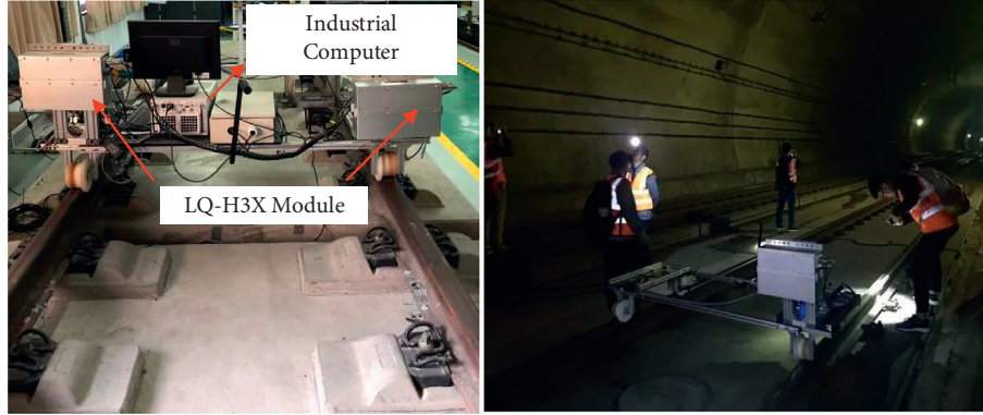
FIGURE 9: Image acquisition. (a) Special rail inspection vehicle. (b) Picture of image acquisition in high-speed railway line.
