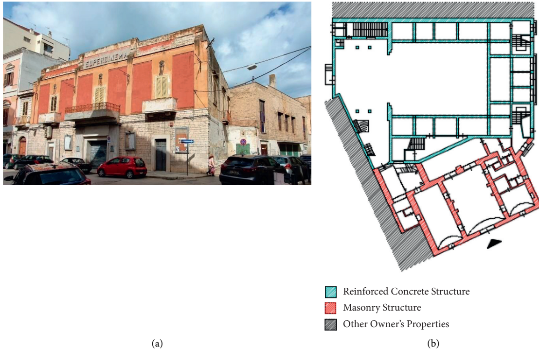
FIGURE 1: The SUPER CINEMA in Trani: (a) front view and (b) structure typologies individuation.
