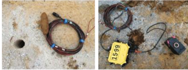
FIGURE 3: Equipment installation at site monitoring points.
