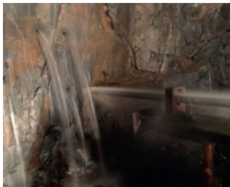
FIGURE 11: Water gushing during advanced drilling.
