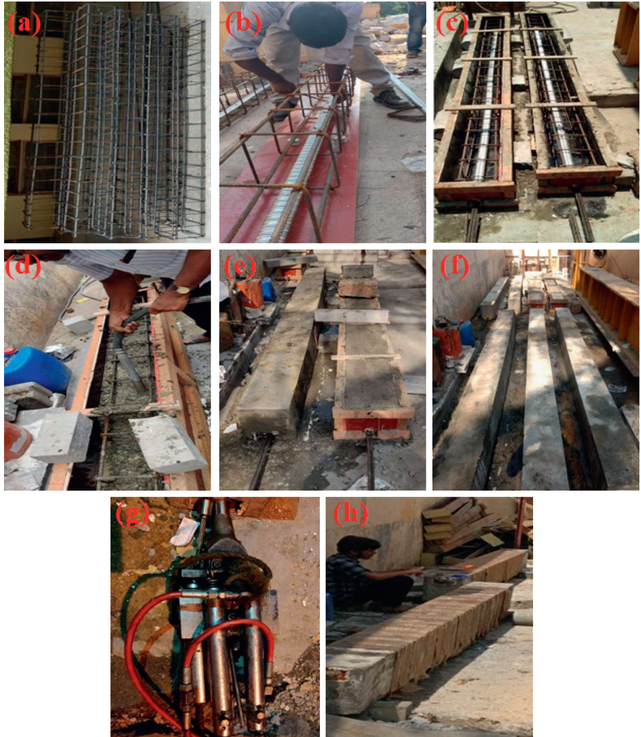
FIGURE 2: Procedure adopted. (a) Steel reinforcement. (b) Anchorage. (c) Sheathing pipe installation. (d) Pouring concrete and compacting with vibrator. (e) Beams to solidify in the mold for 24 hrs. (f) Beams after burr removal. (g) Stressing with hydraulic jack. (h) Jute mat wrap.
