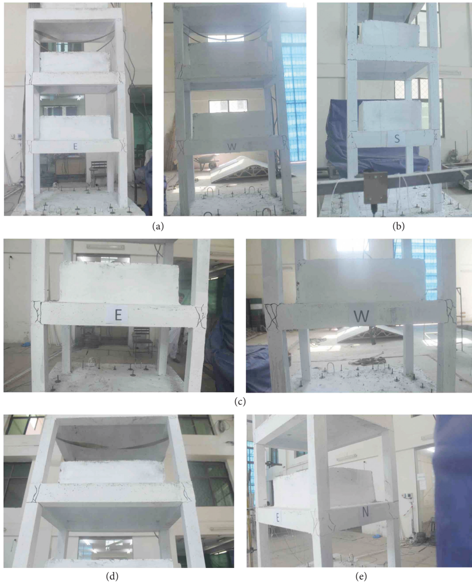
FIGURE 5: Damages observed in the frame structure under 200% earthquake motions. (a) In-plane loaded frame. (b) Face-loaded frame. (c) Damage to joints on first floor. (d) Damages observed in beams and joints at the second floor. (e) Damage pattern at corners.
