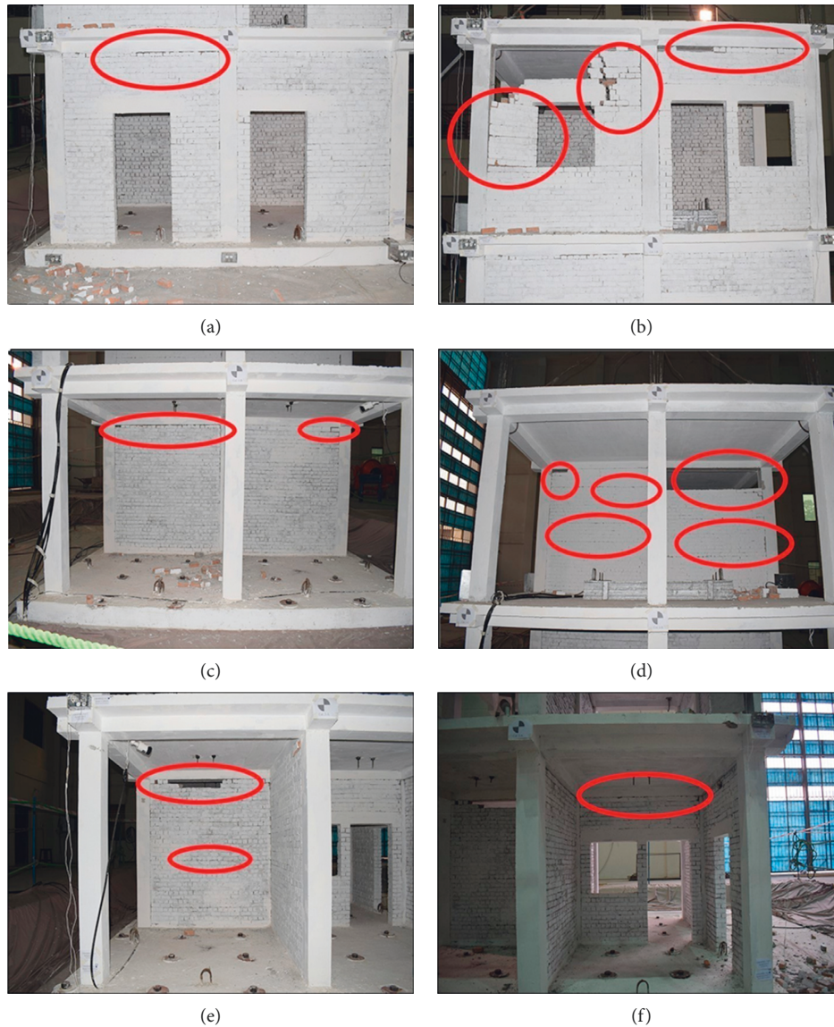
FIGURE 14: Damage observations of URM walls after Test Run-2. (a) Exterior infilled frame of first storey. (b) Exterior infilled frame of second storey. (c) Interior infilled frame of first storey. (d) Interior infilled frame of second storey. (e) Out-of-plane solid infilled frame. (f) Out-of-plane with openings infilled frame.
