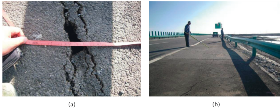
FIGURE 1: Saline soil-induced pavement cracking and settlement.
