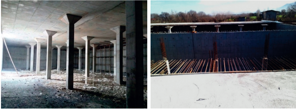
FIGURE 1: Concrete surface tank with 5000 m 3 volume in Kermanshah.
