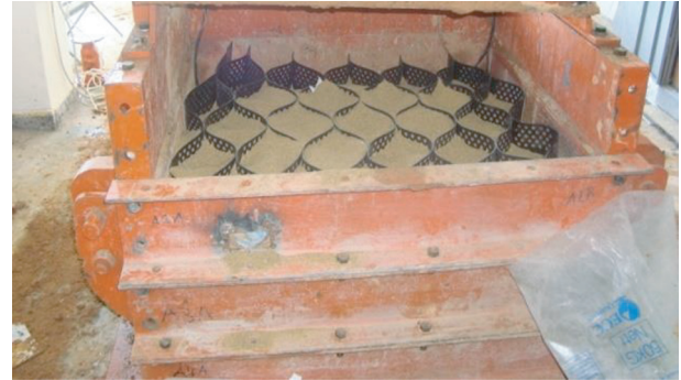
FIGURE 1: Filling the geocell with sand.
