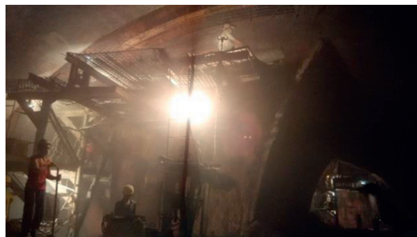
FIGURE 9: Photo of CD method construction in Malin tunnel.
