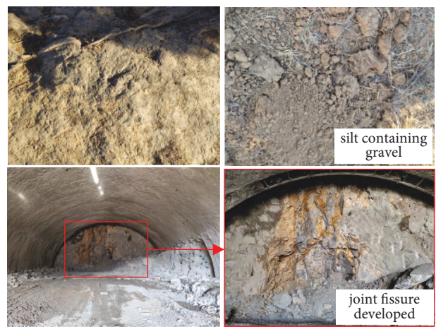
FIGURE 3: Geological features of surface residual soil and surrounding rock.
