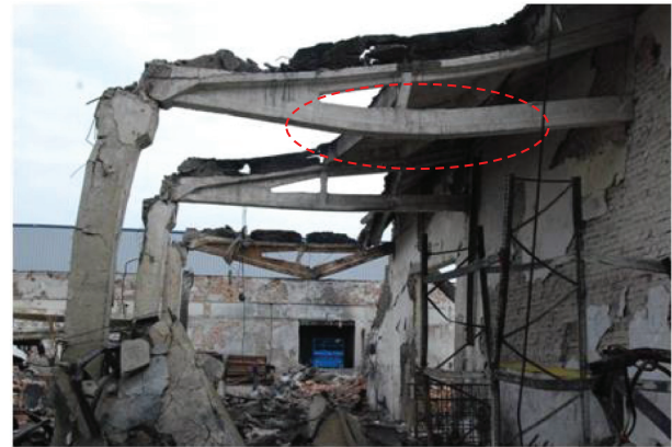
FIGURE 11: Deformation of the centre of the RC girders in a real fire incident [74].
