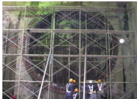
(c) Tunnel eye for launching
