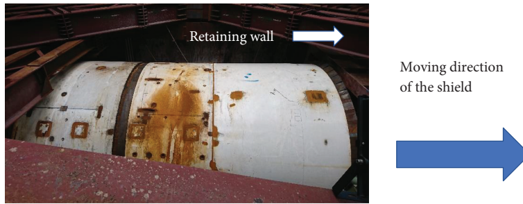
(b) The shield in the pit
