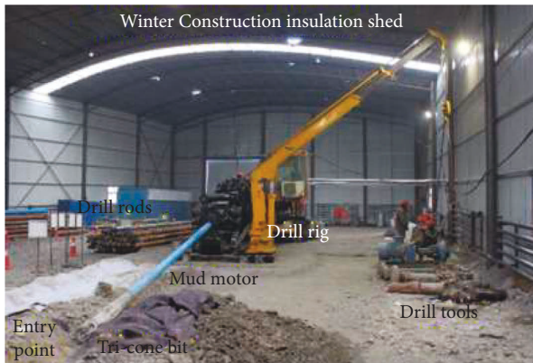
FIGURE 3: Geological survey site of the horizontal directional drilling tunnel.
