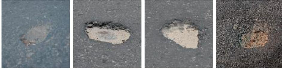
FIGURE 1: Appearances of potholes in the asphalt pavement surface.
