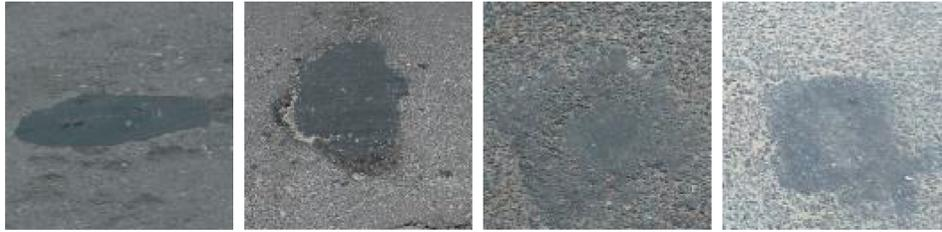
FIGURE 2: Appearances of patched potholes in the asphalt pavement surface.
