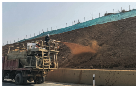
FIGURE 7: External-soil spray seeding.
