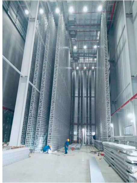
FIGURE 1: High-rise steel pallet racks under construction in China.
