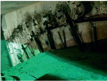
FIGURE 8: Steel sleeve outside the tunnel portal.
