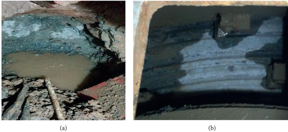
FIGURE 7: Break through plain concrete walls. (a) Drill concrete manually. (b) EPB shield grinding.
