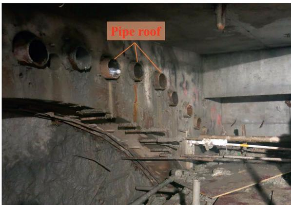
FIGURE 5: Pipe roof installation.
