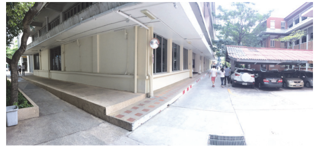
FIGURE 5: Mechanical Engineering Lab.
