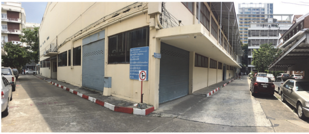
FIGURE 6: Civil Engineering Lab.
