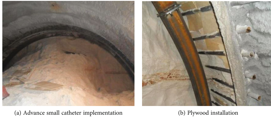
FIGURE 12: The implementation of advanced conduit and plywood installation.
