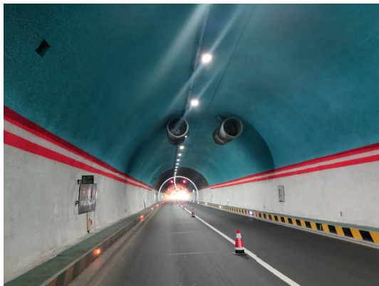
FIGURE 20: Photographs of the operation site of the Dugongling tunnel.
