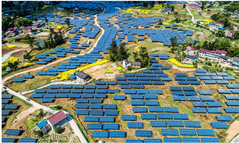
FIGURE 8: Photovoltaic power generation scene in Bade Village, Bashan Town, Zhong County, Chongqing. Chart source: Xinhua News Agency.
