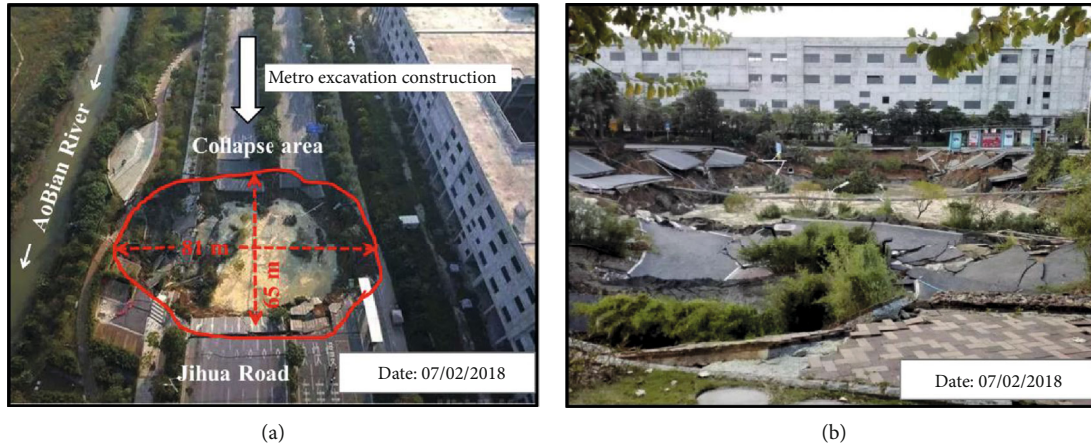
FIGURE 1: Foshan collapse view: aerial (a) and terrestrial (b).
