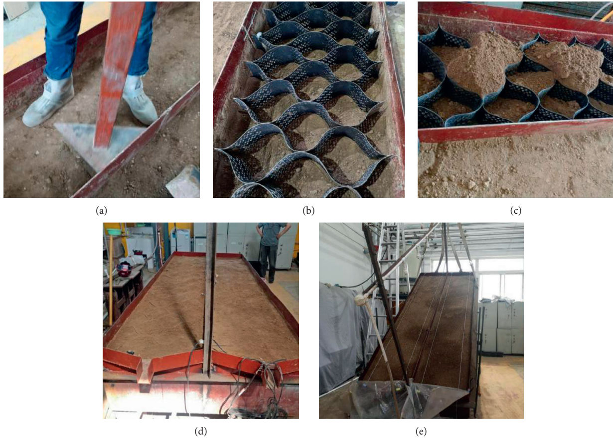
FIGURE 3: Model construction: (a) compaction of base soil; (b) placement of geocells; (c) fill of slope soil; (d) finished model; (e) finished model at a slope ratio of 1:1.5.
