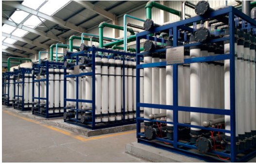
FIGURE 8: Mid-ring membrane thermal ultrafiltration membrane.
