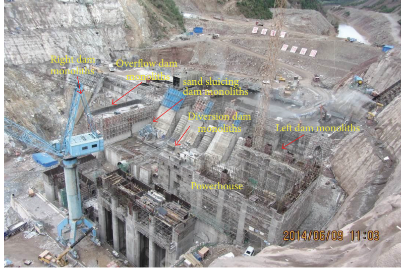
(a) Snapshot of the Guoduo gravity dam under construction
