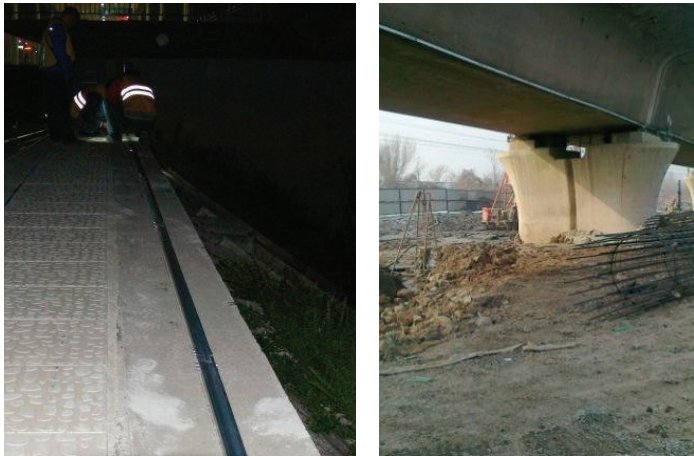
FIGURE 14: Wiring duct layout used in the Beijing-Tianjin and Tianjin-Qinhuangdao high-speed railways.
