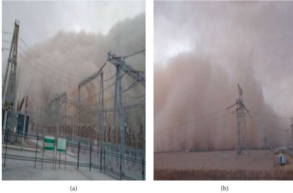
FIGURE 1: Facilities of the power grid subjected to a sandstorm: (a) power substation; (b) tower-line system.
