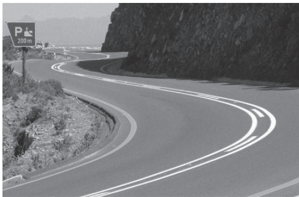
FIGURE 4: Spiral curve in road design.
