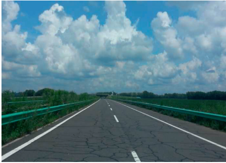
FIGURE 8: Pavement crack in winter.
