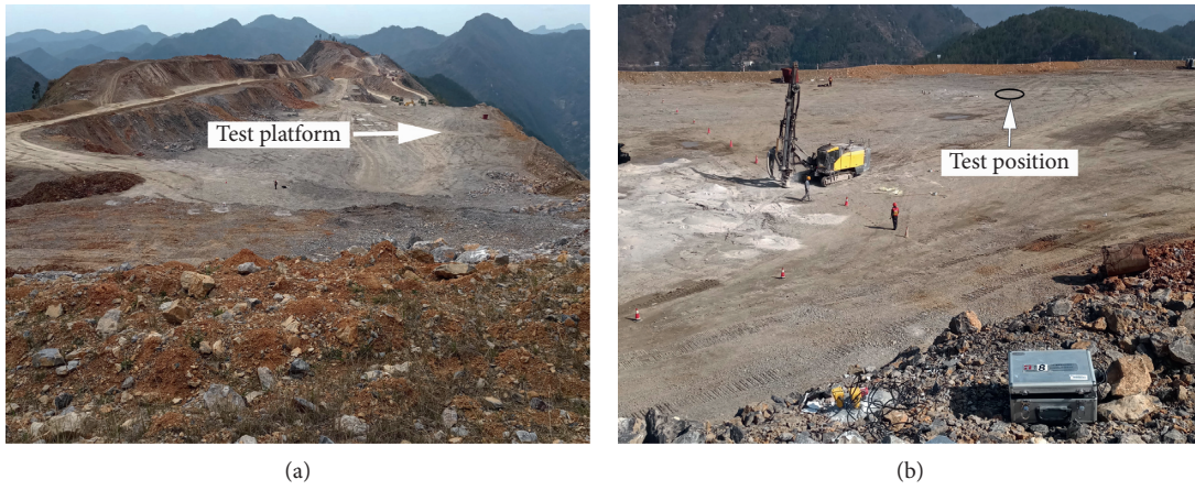
FIGURE 3: Mine test site: (a) test platform; (b) test position.
