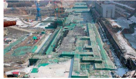
FIGURE 6: Photograph of engineering site of Fengman hydropower station.
