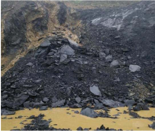
FIGURE 1: Carbonaceous rock slope collapses.
