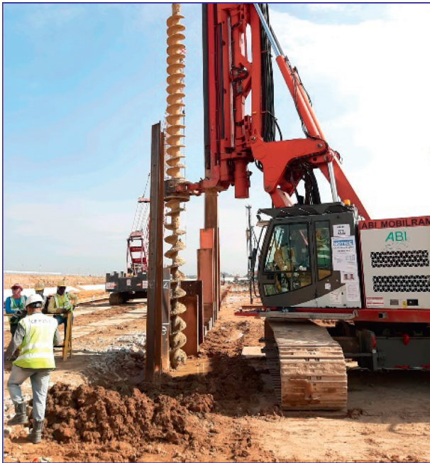
FIGURE 4: Pre-augering process to loosen soil for retaining wall installation.
