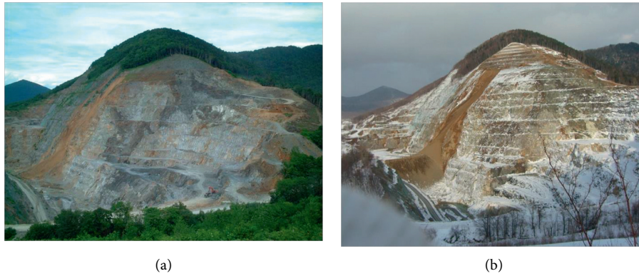
FIGURE 5: Layout of the rock slope (a) before and (b) after cutting upper part of the slope in July, 2004 and November, 2009.
